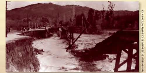
Vineland Avenue being washed out by the North Hollywood flood. View is north from Ventura Blvd.
