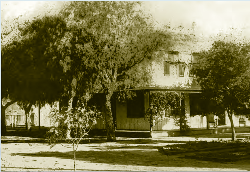
Exterior view of the Lankershim residence.
