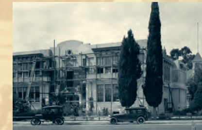
Construction on one of the Lankershim Elementary buildings, located on Bakman Avenue, c. 1920.
