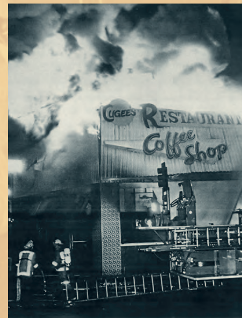
Fully involved structure at Cugee's Restaurant fire after the roof fell and just prior to building collapse.
