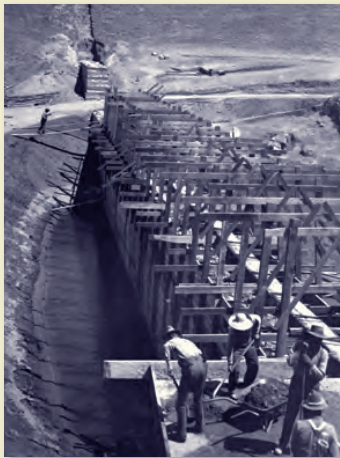
Construction of the L.A. Aqueduct to Owens Valley, between 1907 and 1913. The aqueduct was considered a great engineering accomplishment only second to the Panama Canal.
